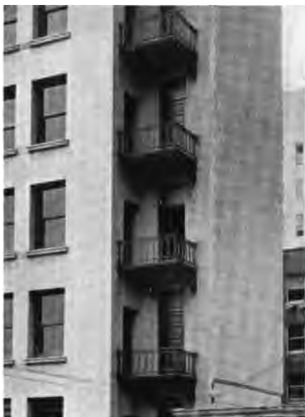
Fig. 1. Balconies leading to Smoke-Proof Tower.*
